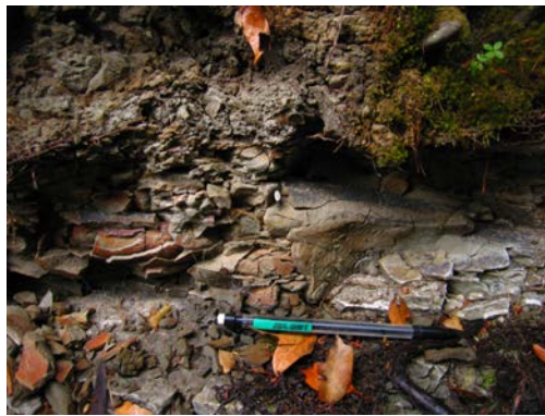
2. Fractured mudstone along the wall of Pescadero Creek, pencil for scale.
